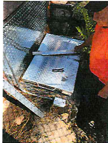
Figure 6 Spring access hatch
