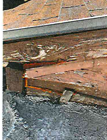
Figure 4 Siding gaps sealed
