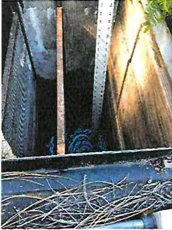
Figure 7 Depth over spring discharge pipe reading
